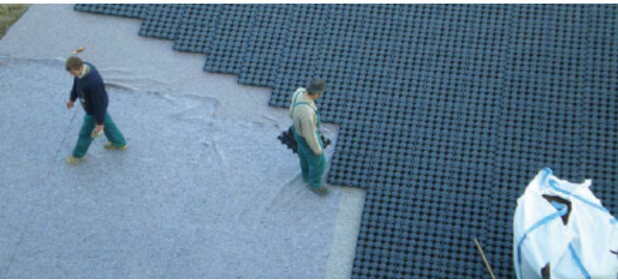
Posa in opera Drainroof
